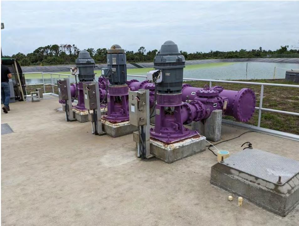
Photo 17: Rotonda WRF Transfer Pumps
