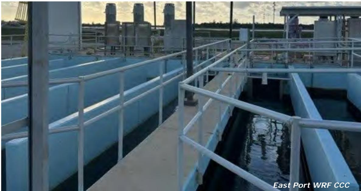
**F. Reuse and Disposal Facilities:** The WRF includes a reclaimed water storage pond that can be used before transmission and distribution through the MRS. In accordance with the reclaimed operating protocol, excess or substandard quality reclaimed water can be diverted to the reject pond or discharged through the on-site sprayfields or deep injection wells.
