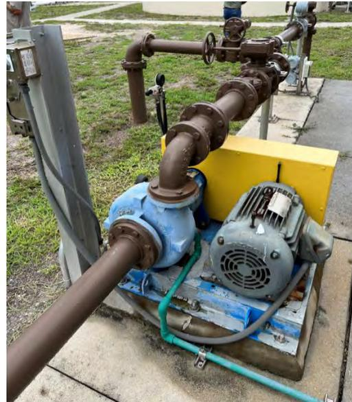
Photo 12: Rotonda WRF RAS Pump    Photo 13: Rotonda WRF WAS Pump
