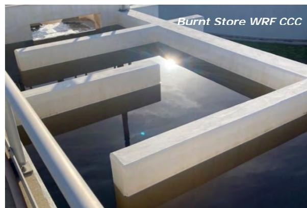
CCC and adjusts the chlorine feed rates. A reagent-less analyzer measures the chlorine residual at the CCC discharge weir for compliance with regulatory limits. Sodium hypochlorite is stored in two tanks with a total capacity of 2,200 gallons.
