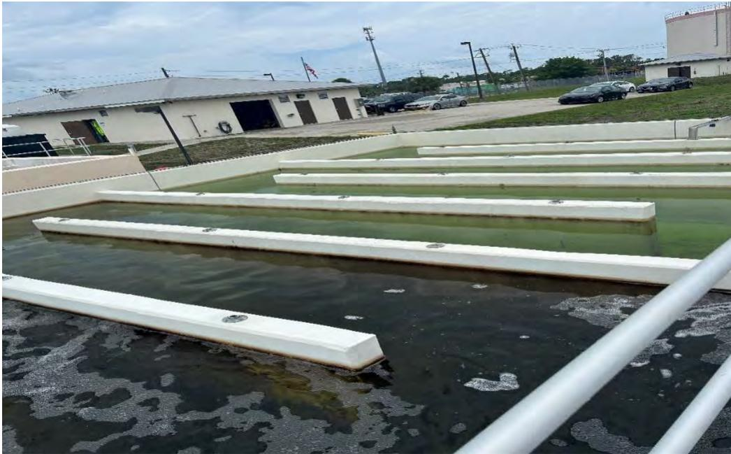
Photo 6: Rotonda WRF Chlorine Contact Basin
