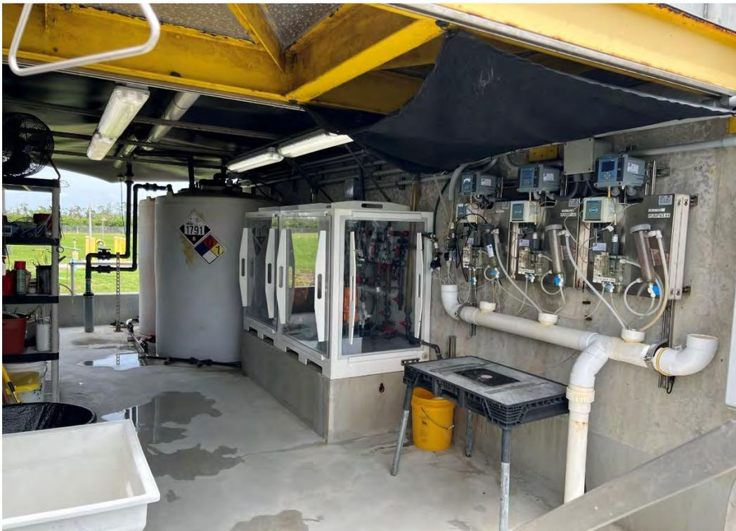
**Photo 28: West Port WRF Chemical Injection System**
