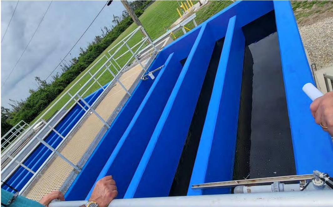
**Photo 27: West Port WRF Chlorine Contact Chambers**
