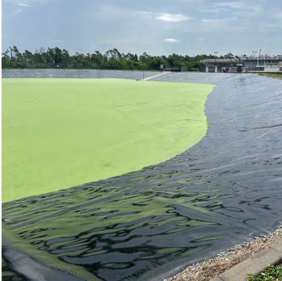
Photo 9: Rotonda WRF Lined Reject Storage Pond
