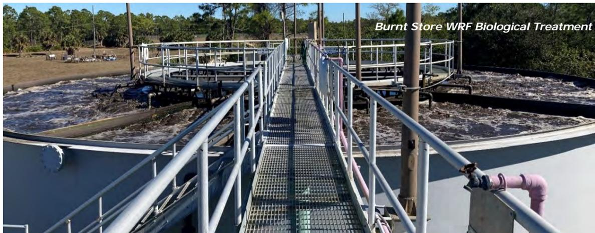
**C. Clarification:** The two steel circular secondary clarifiers are within the center of each package treatment unit for gravity solids separation. The clarifiers are skimmed to remove floatables and scum before clarifier effluent flows over a circumferential weir to the tertiary filters.
