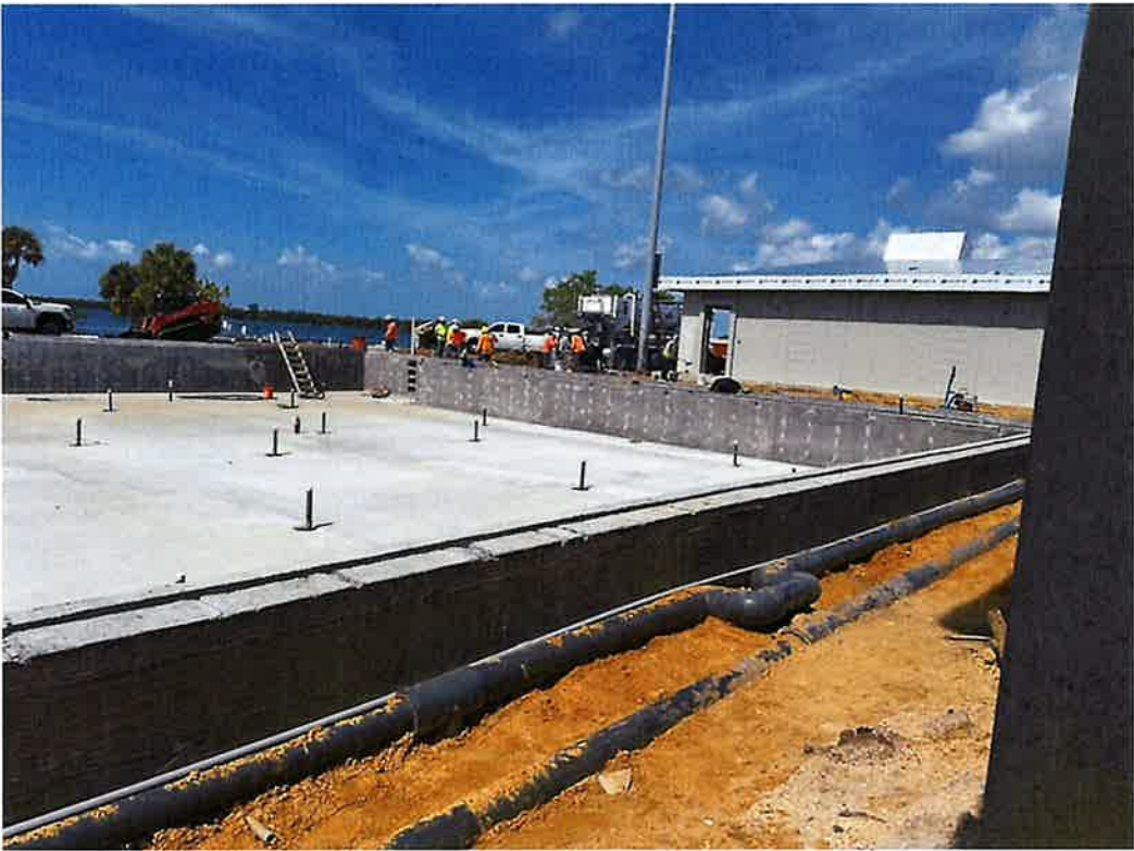
Future Pool in the works.
