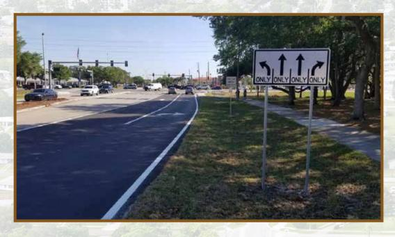
This project consisted of extending the existing right turn lane from Murdock Circle to southbound U.S. 41. The project included new storm drain modifications, construction of the new turn lane along with new signing and pavement markings.
