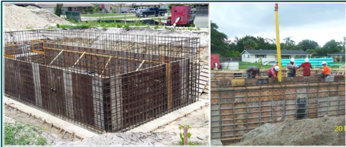
A view of the station foundation base slab and wall reinforcing
