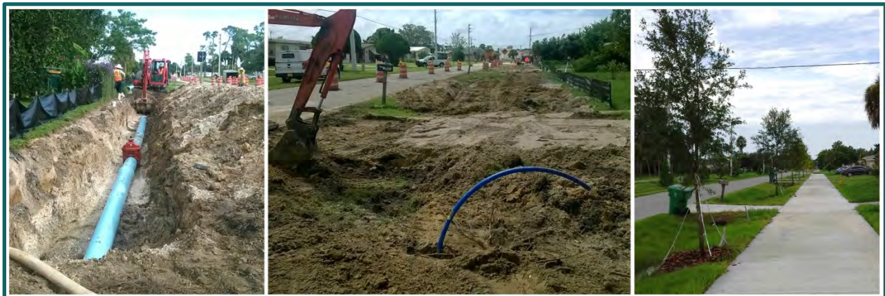
During installation of the pipeline
