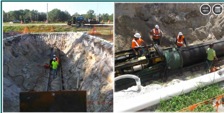
A view of the jack and bore installation at intersection of Ingraham and SR 771. Shown is the carrier pipe that will support the roadway and carry a Utility line.
