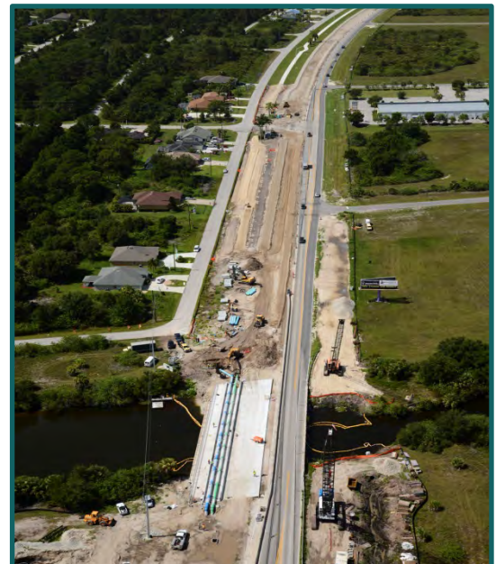
CR 771 Bridge During Construction
