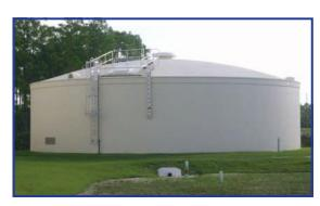
New water storage tanks were part of the expansion of the Burnt Store Water Treatment Plant, completed in 2010. The tanks are capable of holding 500,000 gallons, for the sake of reliability and fire flows.
