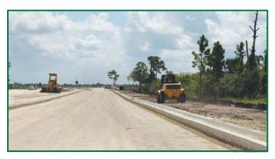
On the Piper Road Project, the curb and gutter is installed before the base material is placed. This step allows for a more efficient work flow, because it is difficult to remove the base material to install the curbing. The curbing also creates a clearly defined space or box for installing the base material in by delineating the road surface and providing a "concrete" (literally) elevation. This material is placed in layers or lifts to ensure that maximum compaction can be achieved.
