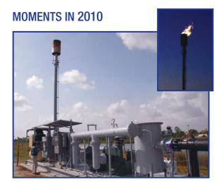
The methane gas-to-energy project at the Zemel Road landfill broke ground in early 2010 and by October Phase I (the flare) was operational. Funded by Mas Energy, the system collects methane the landfill produces and destroys it through a flare (burning) or engines, to be completed in 2011. Both Charlotte County and Mas Energy will receive ongoing revenue from the sale of energy and carbon credits, with the County's portion estimated to be \$800,000 per year.
