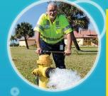
The Charlotte County Utilities Department will flush hydrants only when required. This normally occurs to maintain disinfection residual, to correct taste or odor issues, for service or repair of water mains, or as part of fire hydrant testing and maintenance. Hydrant flushing may occur even during instances of severe water conservation if testing indicates it is necessary for healthy water.
