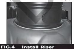
**STEP 4** Screw the riser into the tank joint, being careful that the gasket remains in position. Properly installed, the gasket should show uniform compression around the entire joint. (Fig.4)
