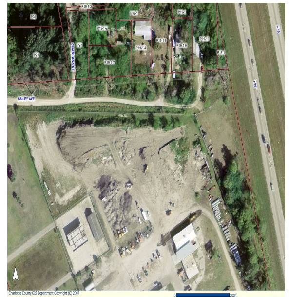
Aerial view of the scale house location at the landfill
