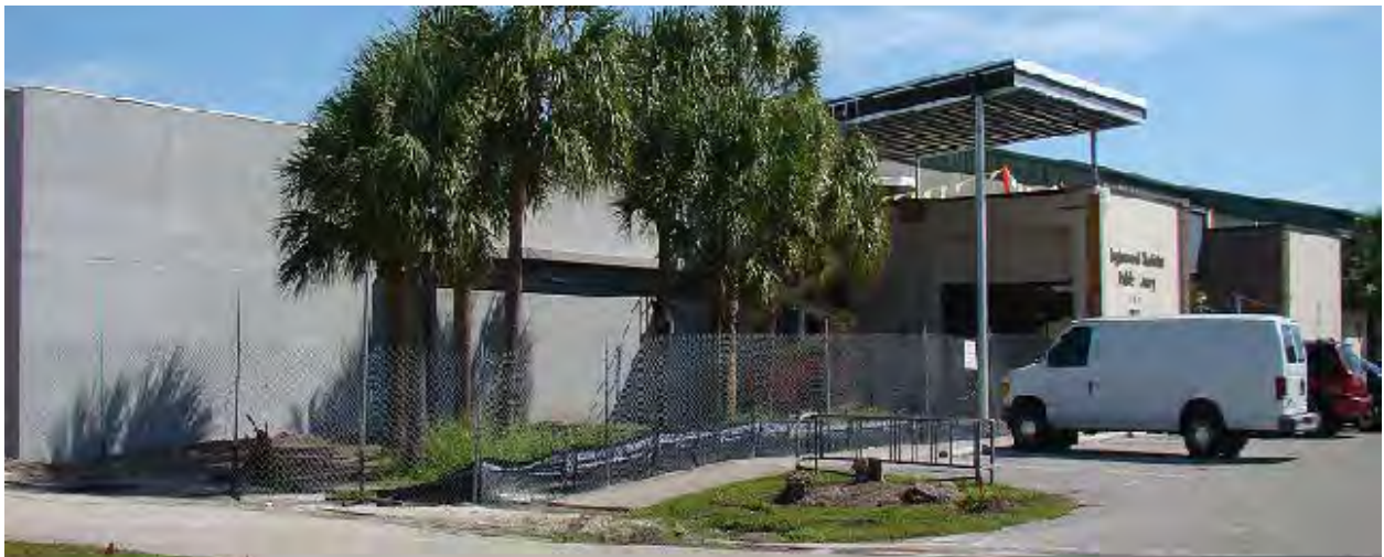
Englewood Library Expansion
