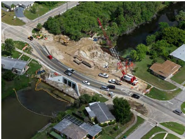
Midway Stormwater Control Structure
