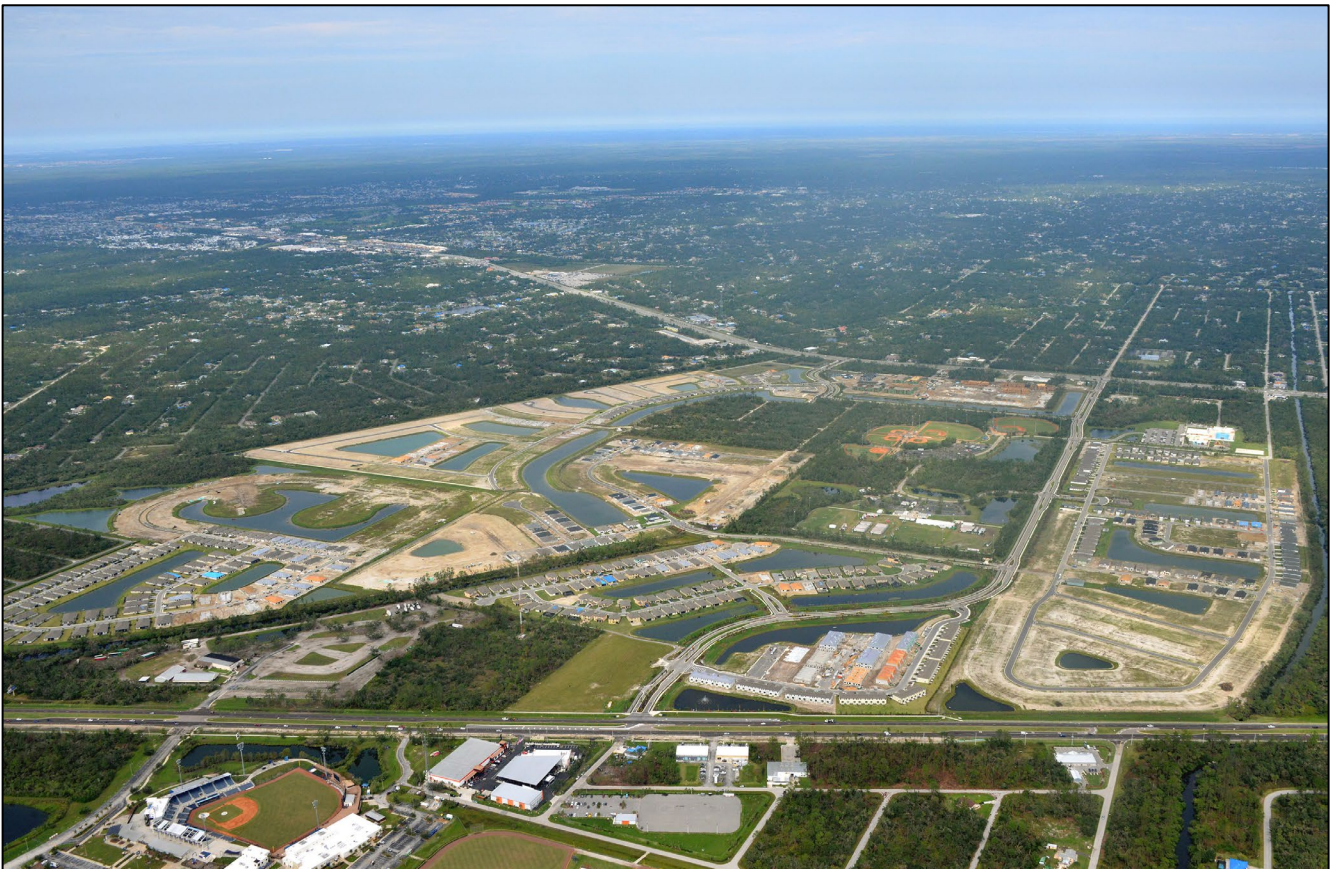
Figure 3 - West Port Phase I Progress, November 2022
