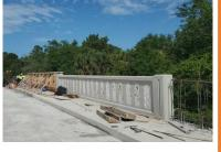
Blvd. over the Markham Waterway, between McDill Dr. & Ramblewood St. in Northwest Port Charlotte. This project will include necessary bridge repairs as noted in the FDOT Bridge Inspection Report, which includes updating the bridge to current design codes, bat exclusion, and Charlotte County utility relocation.
